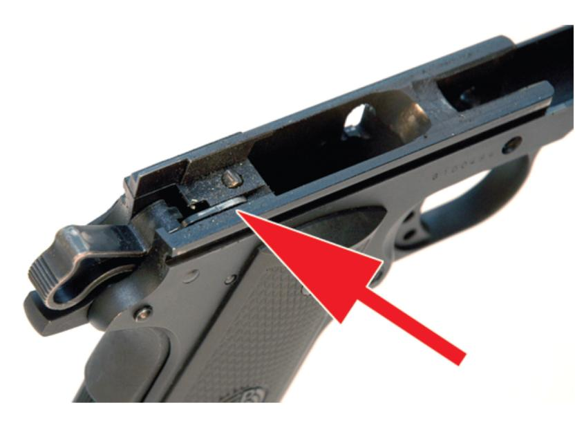
shown to the right of the disconnector (arrow) released the firing pin by pushing upward on a plunger mounted on the bottom of the slide.
